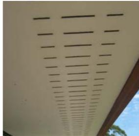
Slotted Hardiflex soffit sheeting
