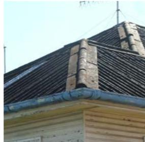
Super Six roof sheeting and guttering
