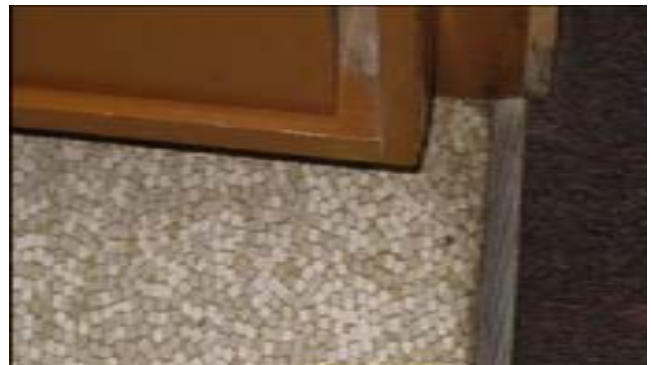
Figure 2 – Terazzo type asbestos backed vinyl sheet flooring.
