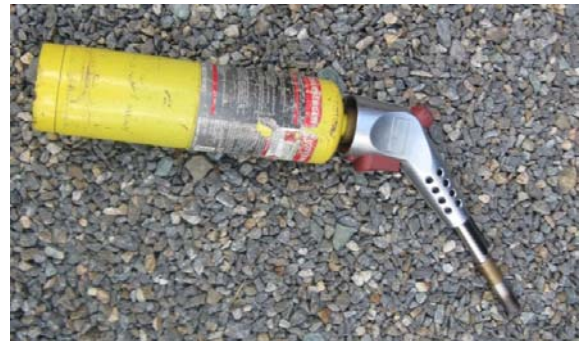
Photograph 2: The welding torch fitted to the disposable MAPP gas cylinder.
