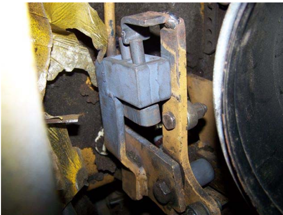
Photo 4: Showing a modified mechanical interlock arrangement controlling the engagement of both the reverse and forward gear shift mechanism.
