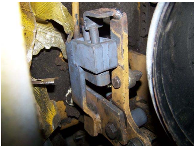
Photo 4: Showing a modified mechanical interlock arrangement controlling the engagement of both the reverse and forward gear shift mechanism
