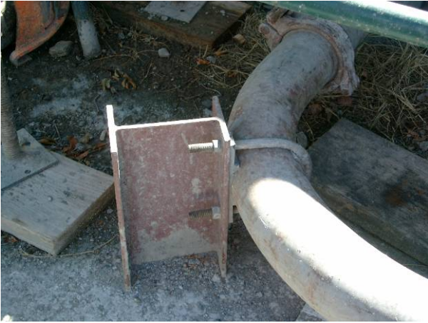
Figure 2. One method of anchoring pipe.
