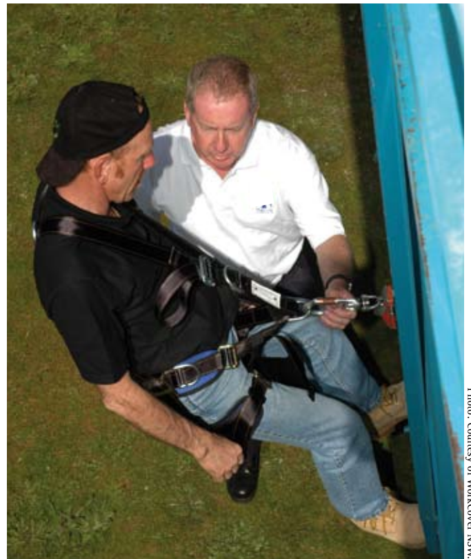
An example of a fall arrest system.
