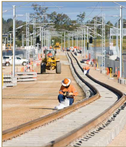
A Queensland Rail construction site
