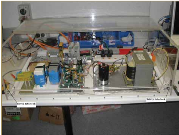
The LV test box
