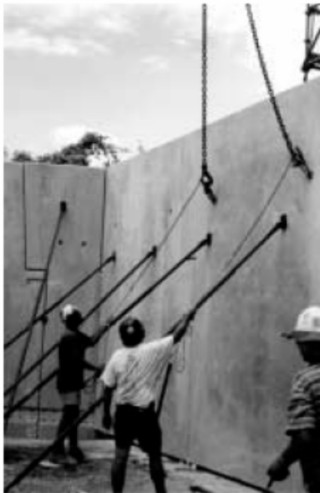
Diagram 9 – Lifting clutch release lines
