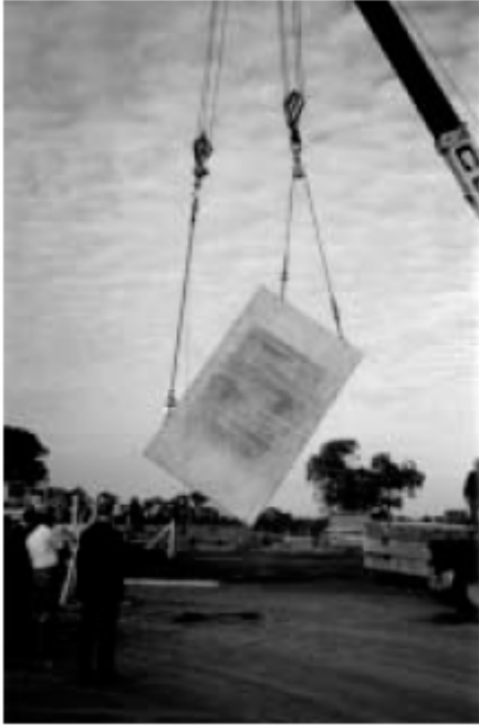
Diagram 11 – Rotation of a pre-cast panel
